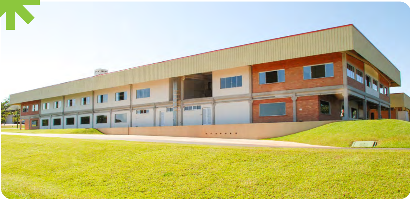
Social building – Itaberai.
